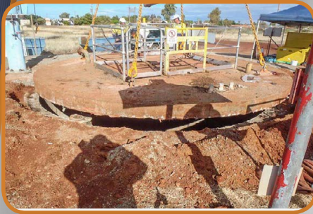
Removing Top Slab
