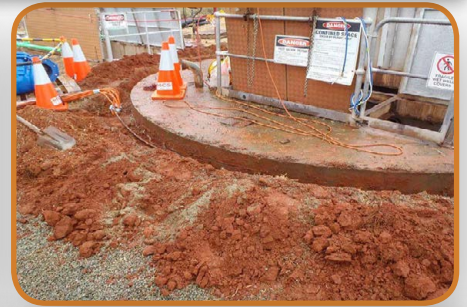
Excavate Around Slab For Removal
