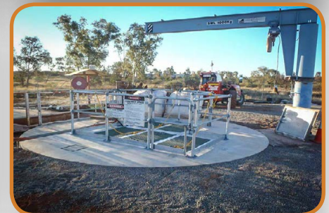
New Top Slab In Place
