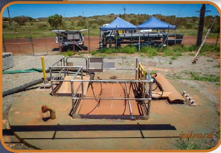
Existing Top Slab In Place
