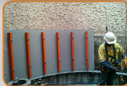
Start Plastic Lining At Bench Level
