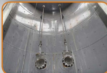
Pipework and Fittings Replaced
