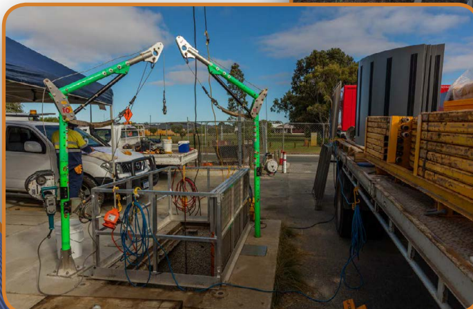
Confined space system setup for access chamber entry
