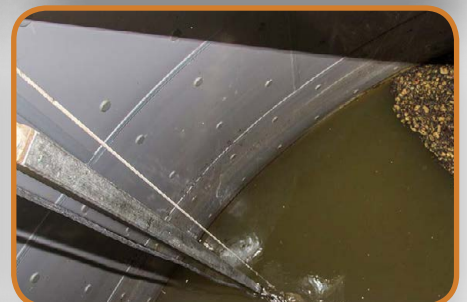
Back In Operation
