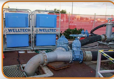
Bypass Pumping Operating
