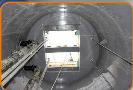
Plastic Lining Completed
