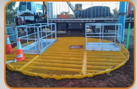
Install Steel Mesh Safety Cover
