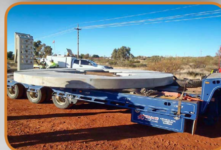
New Plastic Lined Top Slab
