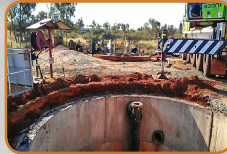
Top Slab Removed
